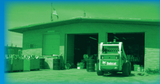
Northfield Township Road District Garage 1928 Lehigh Ave., Glenview
